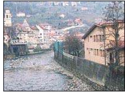
Rossiglione's school (right) has been rebuilt from the ground up
